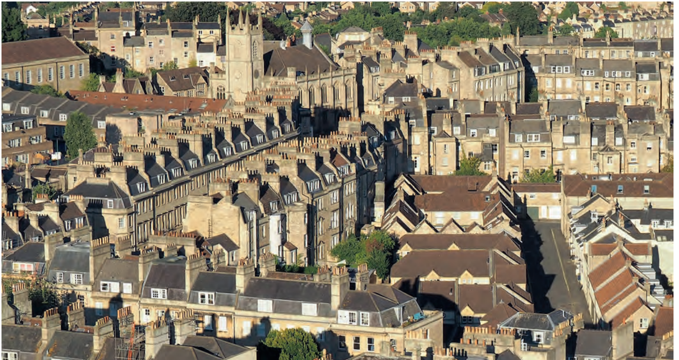
Georgian Bath: increasing levels of insulation could lead to a rash of roof vents across the historic roofscape, but would they reduce condensations? (Photo: Jonathan Taylor)
