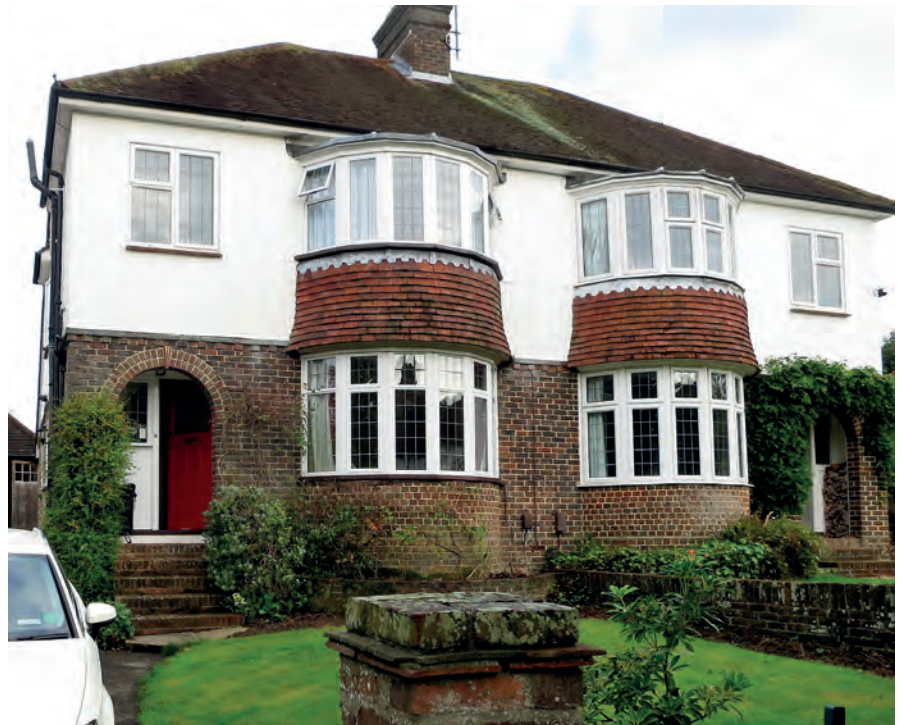
Monitoring the interior environment of the roof of a typical semi-detached house showed that its humidity levels naturally followed conditions outside: contrary to popular belief, increasing ventilation would not affect its ability to dry. (Photo: Brian Ridout)
