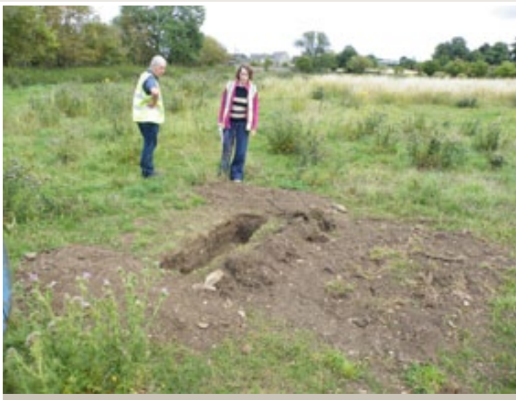
Left: Sarah Bridges of Northamptonshire County Council inspecting damage at Chester Farm © Northamptonshire County Council
